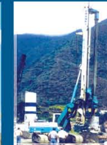
Pilas Circulares Diam.: 0.45 - 2.00 mts. Prof. max.: 40 - 50 mts.
